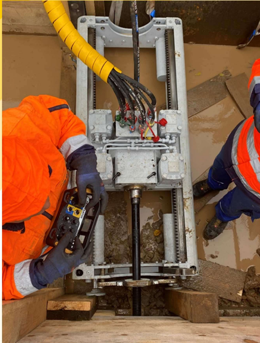
TAIFUN 15 – horizontal directional drilling (HDD)
